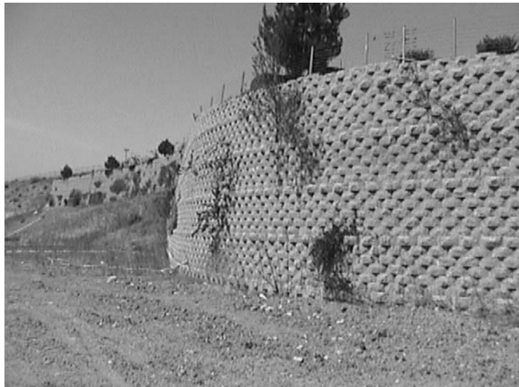
Photo 1 – Geogrid Mechanically Stabilized Earth Wall
