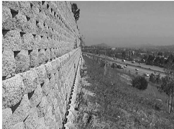
Photo 2 – Close-up of Geogrid Wall
